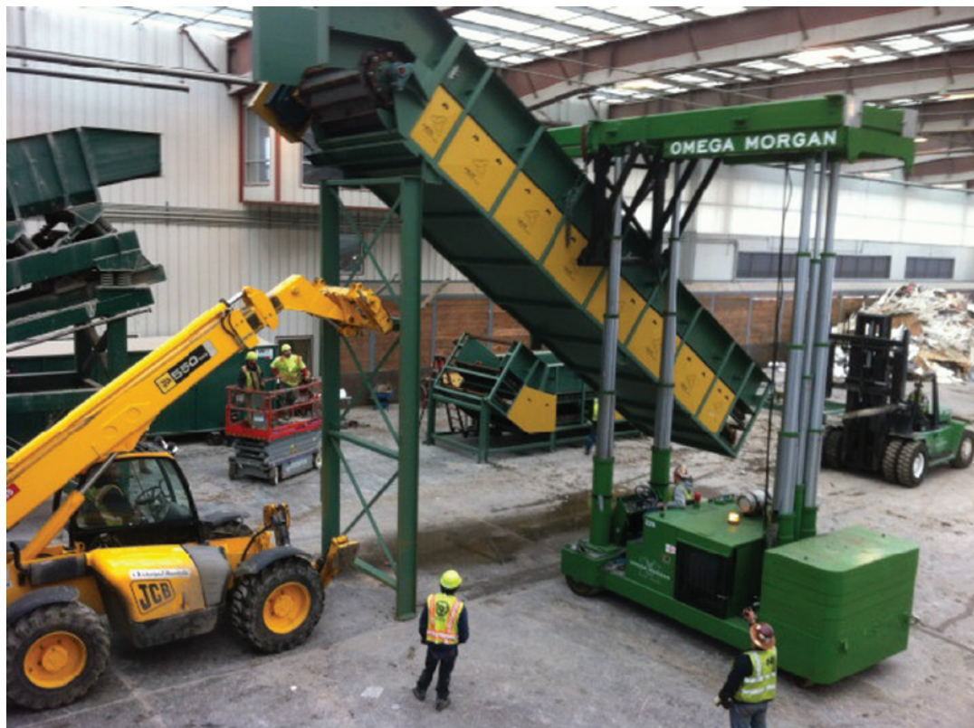
Infeed conveyor retrofit for C&D. Photos courtesy of OEM Sherbrooke.
